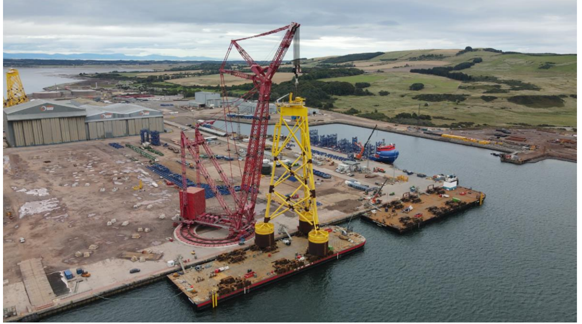
Massive offshore wind platforms need equally massive cranes
